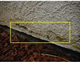
Re-direct spray as required as chronic wetness can cause finish and moisture barrier damage and other moisture problems.
