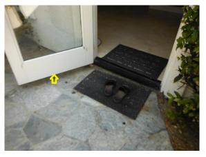
When an exterior door opens outward, there can only be a max 1" distance to the landing (distance between the top of the threshold and landing surface on the exterior). It's possible that these doors were all originally designed open inward but were altered during the actual construction.
