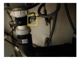
Technically, this is a prohibited cross connection between grey and potable water and is not allowed. Recommend creating an air gap to eliminate this potentially unsanitary condition. A licensed plumber who has experience with reverse osmosis systems may be able to make recommendations for correction.
