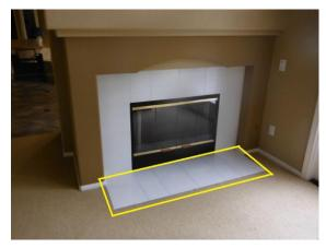
\* The fireplaces show some sooting of the artificial logs and refractory panels. Sooting indicates incomplete gas combustion. One result of incomplete combustion is the formation of, at least, a small amount of carbon monoxide gas. Recommend the gas log set be examined to assure proper burn/combustion.
