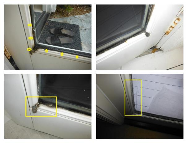
It's possible that the thermpane glazing was replaced in these doors and was not reinstalled well. Our concern is that water will be able to get behind the millwork/trim and eventually damage the doors.
