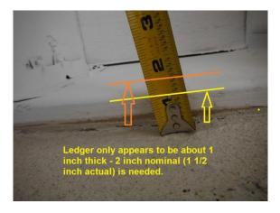
The ledger board is required to be of naturally disease resistant wood, e.g., redwood or pressure treated wood that could typically be identified by the incising (indents). We have no visual evidence that it meets either naturally disease resistant wood or pressure treated wood.
