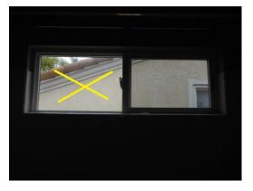
For any failed thermopane windows, the only correction is replacement of the sealed glass unit. Recommend that a qualified glazing contractor review the status of all thermal pane glazing to confirm its status and cost replacement before the release of contingency.
