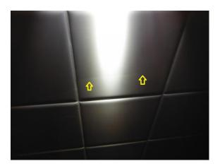
Indent cracks, typically, indicate some workmanship errors with installation of subsurface materials, for example, failure to a properly tape a joint between two sections of backer board (water proofing board) or differential drying shrinkage where there are different thicknesses of the mortar/brown coat/adhesive applied behind the wall for the purpose of attaching the tile to the backer board.
