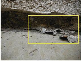
Direct, visible **foundation/structure appear intact and performing as intended.** The areas where we are able to view the edge of the foundation slab revealed no indicators of problems.
