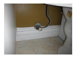
Most of the flexible, metal water supply connectors serving the plumbing fixtures are obsolete. A failed water connector can lead to extensive flooding/damage. As an improvement, recommend replacing the obsolete connectors with braided stainless steel connections which are far less prone to fail over time.
