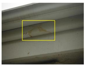
While this most likely reflects water flow behind the gutter which reflects some gutter system shortcoming, we cannot rule out the possibility that water is getting under the tiles above this area and coming out at the bottom of the shadow board. We recommend that a licensed, competent roofer confirm the exact situation/conditions and make any recommendations for correction/repair ideally before the release of contingency.
