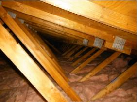
Roof trusses are an assembly of wood pieces (most often 2x4 dimensional lumber) connected together with steel plates to form a unified structural member.
